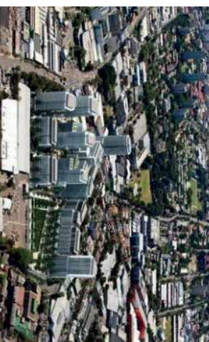
Fig. 76.41 Aerial image of Green Square development Source: Arup, 2018
