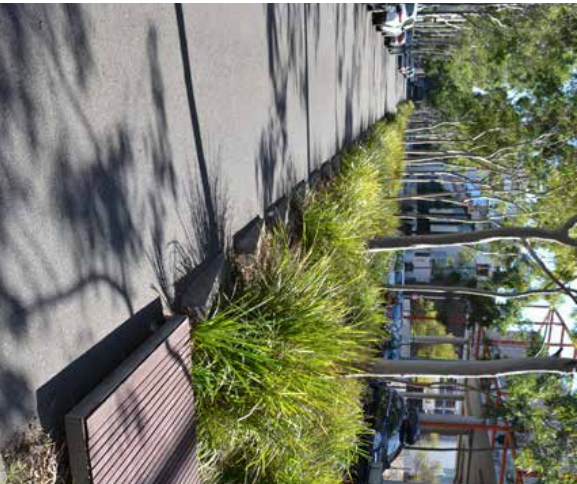
Fig. 7.6.65 Integrated bio-drainage Source: Architecture Au
